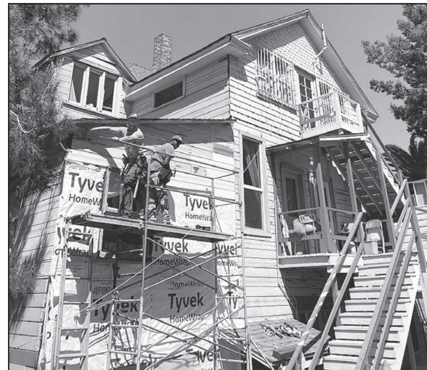
Kaleb and Bert work on Hennacy House renovation project
